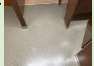
New Flooring and Partitions
